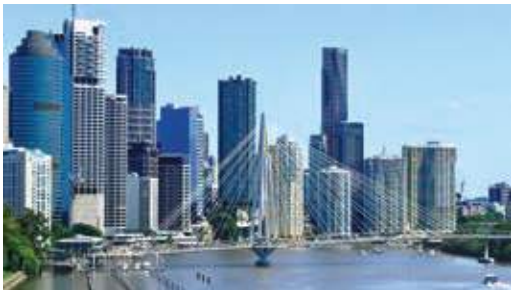
The Kangaroo Point Bridge, a project under the Brisbane City Plan, opened in December 2024 with dedicated paths for pedestrians and cyclists 439 Photo courtesy of Chris Olszewski (CC BY-SA 4.0) / Wikimedia Commons
