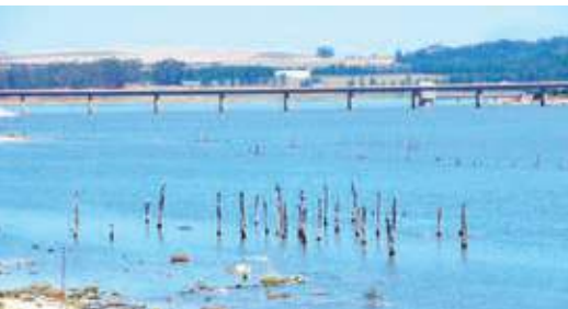
Theewaterskloof Dam in South Africa is one of the key dams supplying water to Cape Town 434 Photo courtesy of Olga Ernst (CC BY-SA 4.0) / Wikimedia Commons
