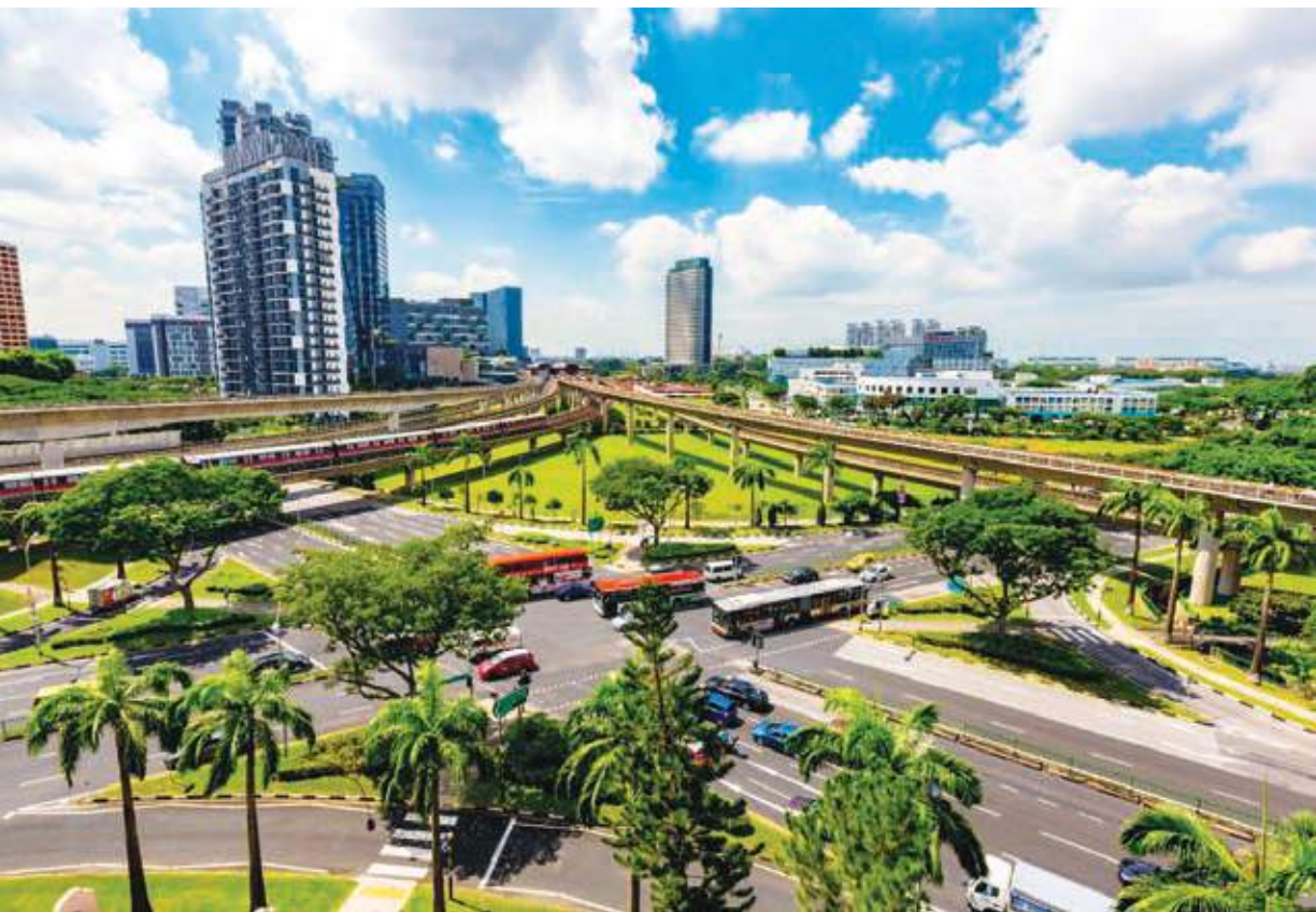
The effectiveness of integrating land use planning and mobility can be seen in the example of Jurong East Photo courtesy of Land Transport Authority
