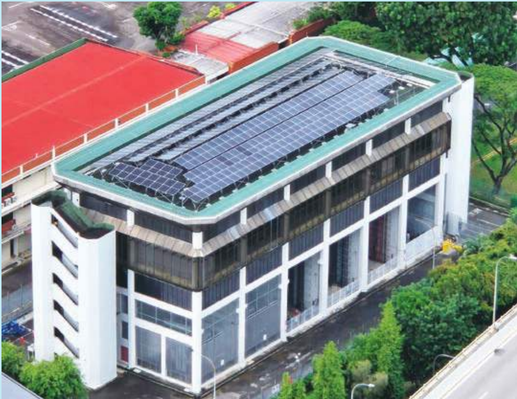
SP Group has deployed rooftop solar panels on substations island-wide, with a total installed capacity enough to power more than 4,500 four-room HDB flats for a year Image courtesy of SP Group
