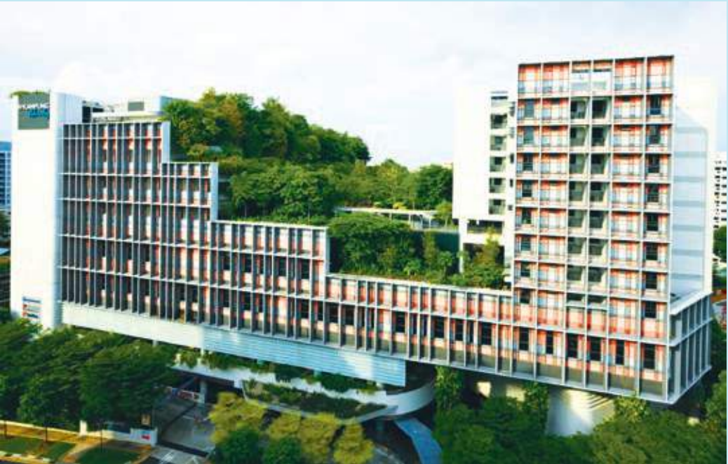
Kampung Admiralty is an integrated development with apartments for the elderly that are co-located with a medical centre, facilities for childcare and eldercare, and green spaces
